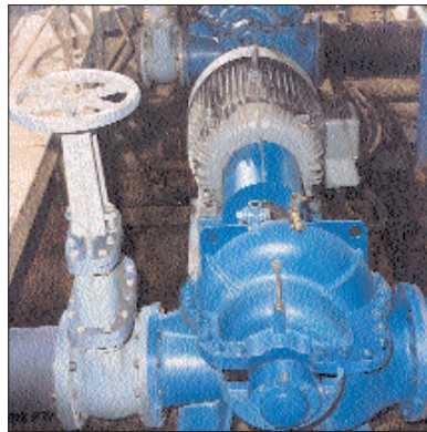
A split case cooling circulation pump
