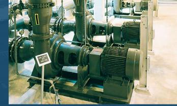
The Morris 7100 is a series of large dry-pit pumps that can handle abrasive solids. A long service life and efficient operation are assured by robust materials, thick cast casing and customized design. The impeller and casing design ensures smooth vibration-free pumping.
