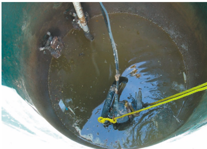
Top view showing Upgrade retrofit.
