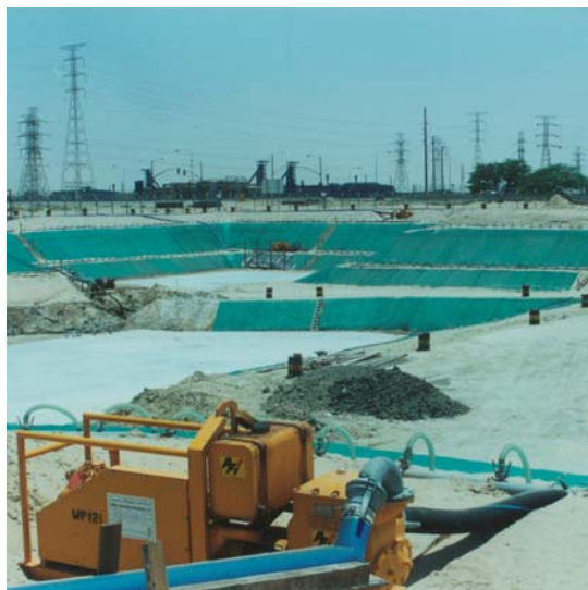
Wellpoint dewatering at sewer and storm water drainage lines and oil and gas pipelines.
