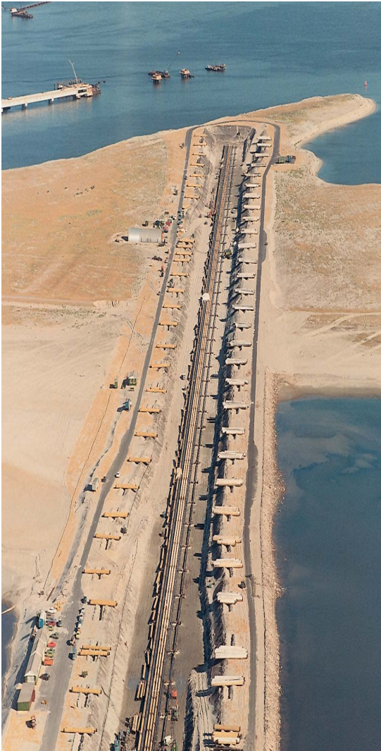
Excavated dry dock for 12-pipe bundle.
