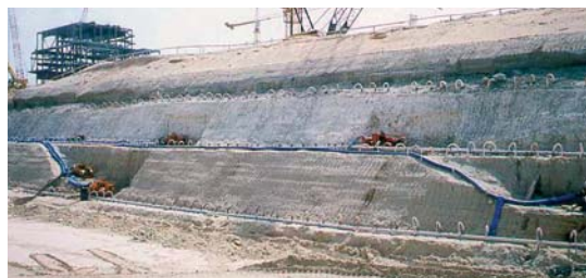
Three-stage vacuum wellpoint system at a 15 m deep excavation.
