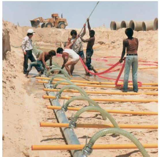
Wellpoint placing with jetting pipe.
