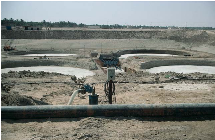
Deepwell dewatering underground storage tank site.
