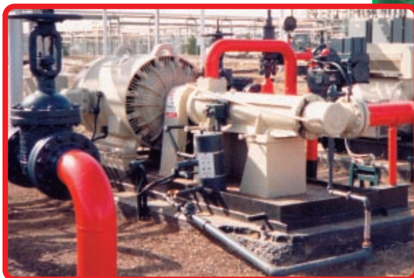
12D-400P on crude oil pipeline service in Alberta, Canada at 1440 PSIG (99 BAR)
