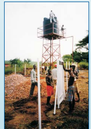
Community members setting up a fence and overhead tank for the SolarPedalflo.
