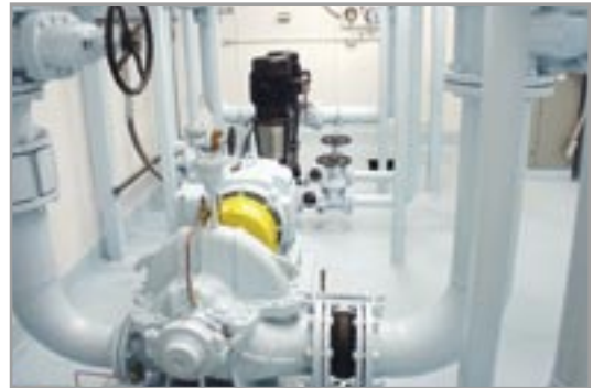
Above Ground Installation.
