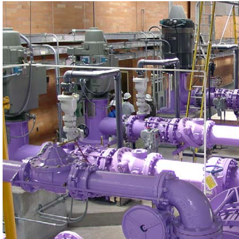
Left: Water re-use pumps Below top: Field installation Below bottom: Booster pumps
