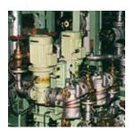
Pump: KF 74. Medium: HFO, MDO. Delivery rate: 20 to 74 I/min.
